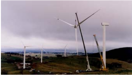
Erection of wind rotor and massive crane assembling a tower at the Blayney Wind Farm
