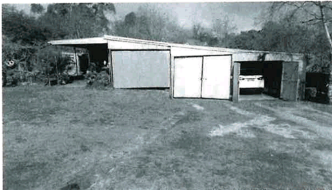
General view of the existing shed from the rear yard
