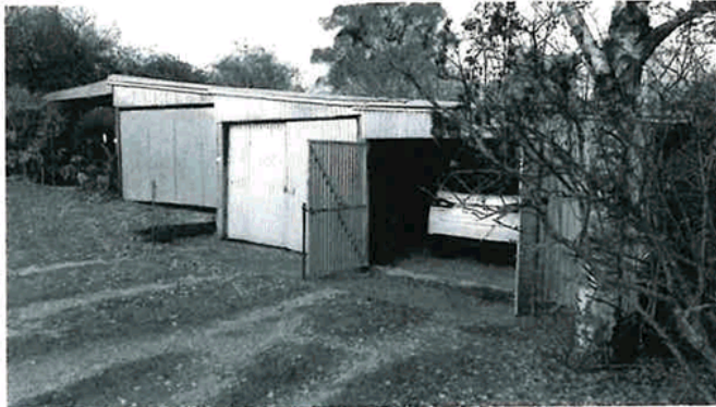
Close view of the existing shed to be replaced
